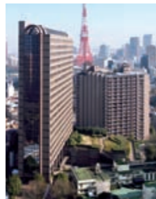
ROPPOHGI FIRST BUILDING / ROPPOHGI FIRST PLAZA / ROPPOHGI VIEW TOWER
