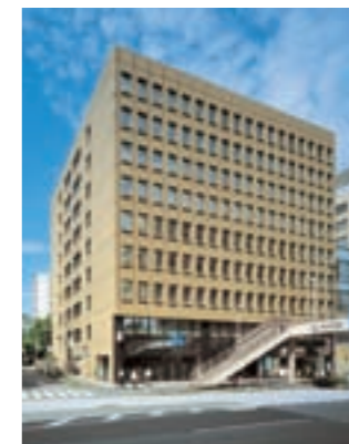
TORANOMON 35 MORI BUILDING
