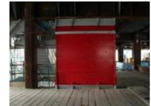
Viscous seismic damping wall
