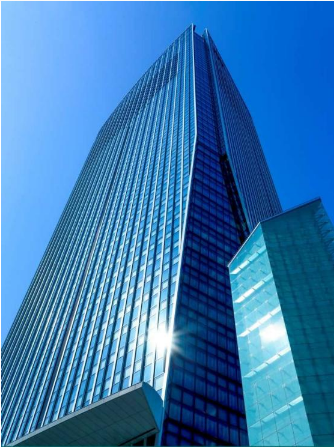
Toranomom Hills Mori Tower
