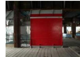
Viscous seismic damping wall
