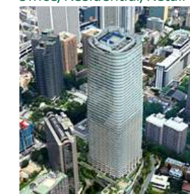
ARK Hills Sengokuyama Mori Tower
