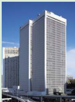
ARK Mori Building
