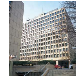
Toranomom 37 Mori Building
