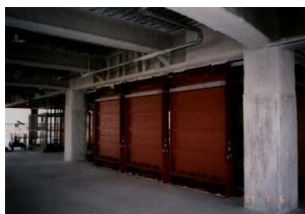
Viscous seismic damping wall
