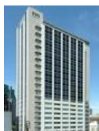
Holland Hills Mori Tower
