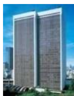
ARK Mori Building
